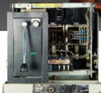
Pre-Engineered Retrofit Solution Upgrade E&A CNCS ACB to OMEGA ACB
